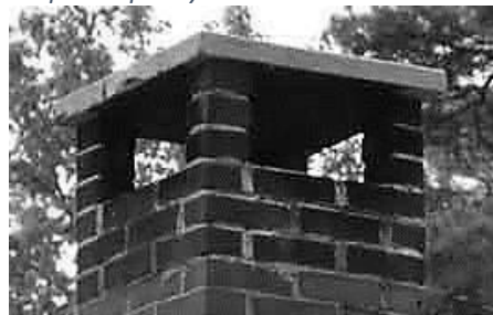
Concrete Cap Chimney Top
